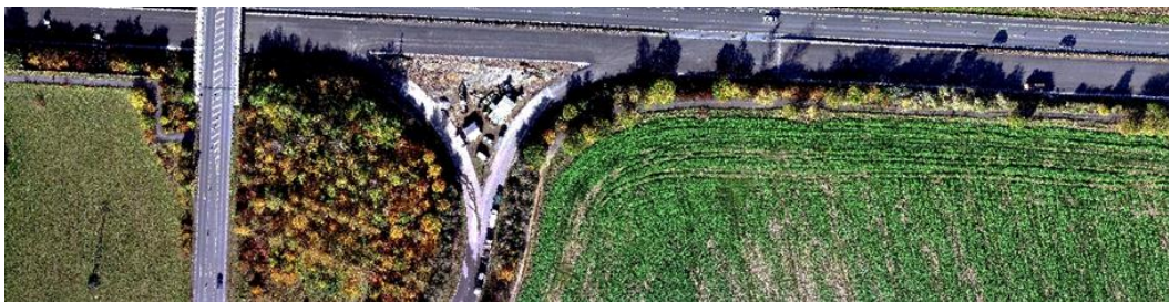
Fig. 5 Vertical view of orthophoto mosaic of D6 motorway section, source: own
